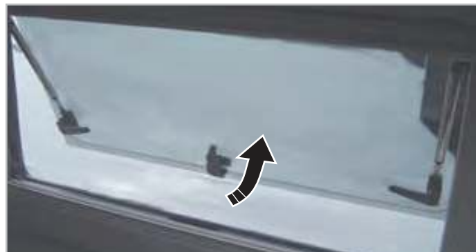
Fig.6.3 - Opening the windows
